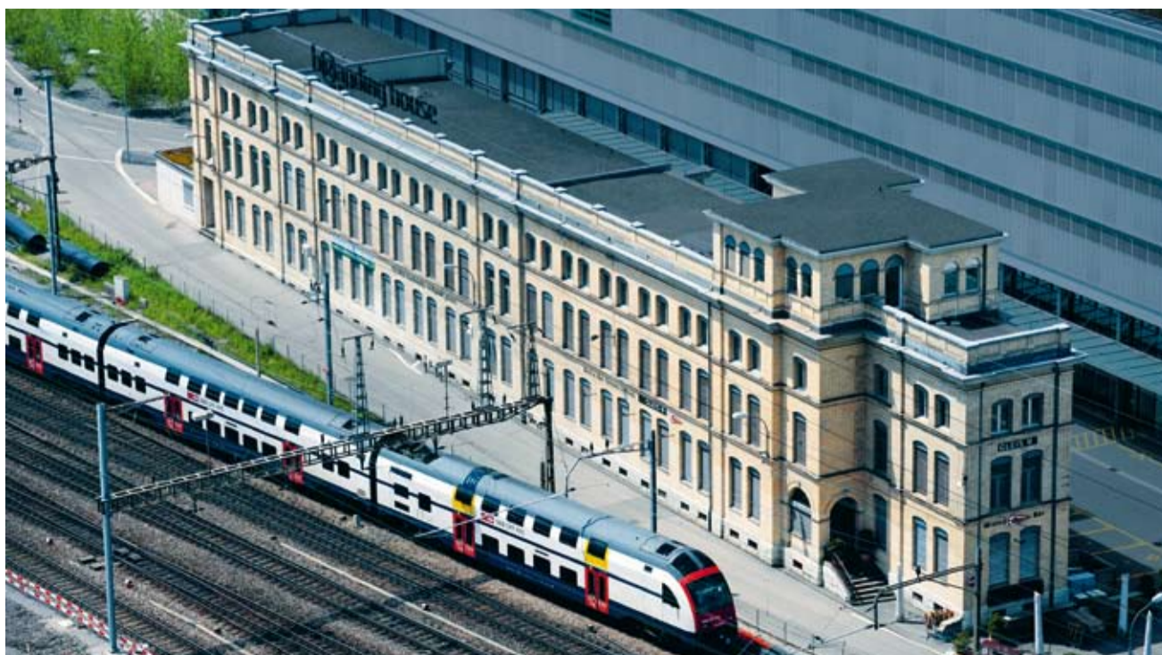
The 6200-ton-heavy MFO building will be relocated 60 metres to the west on rollers in March 2012.
